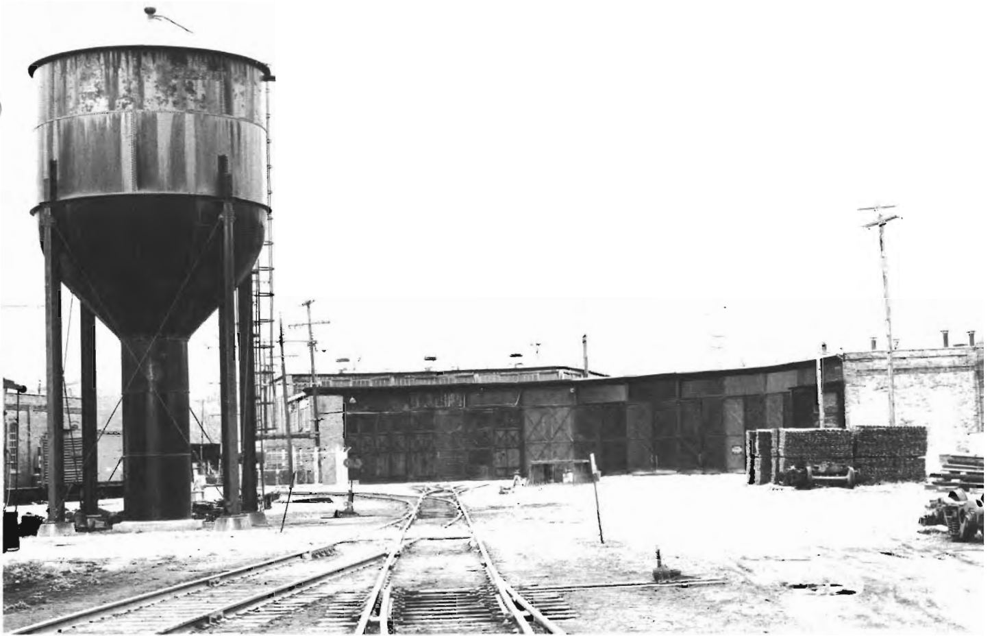
Above - One of only two roundhouses left on the DT&I, this one, at Jackson, is now used by the car shops.
