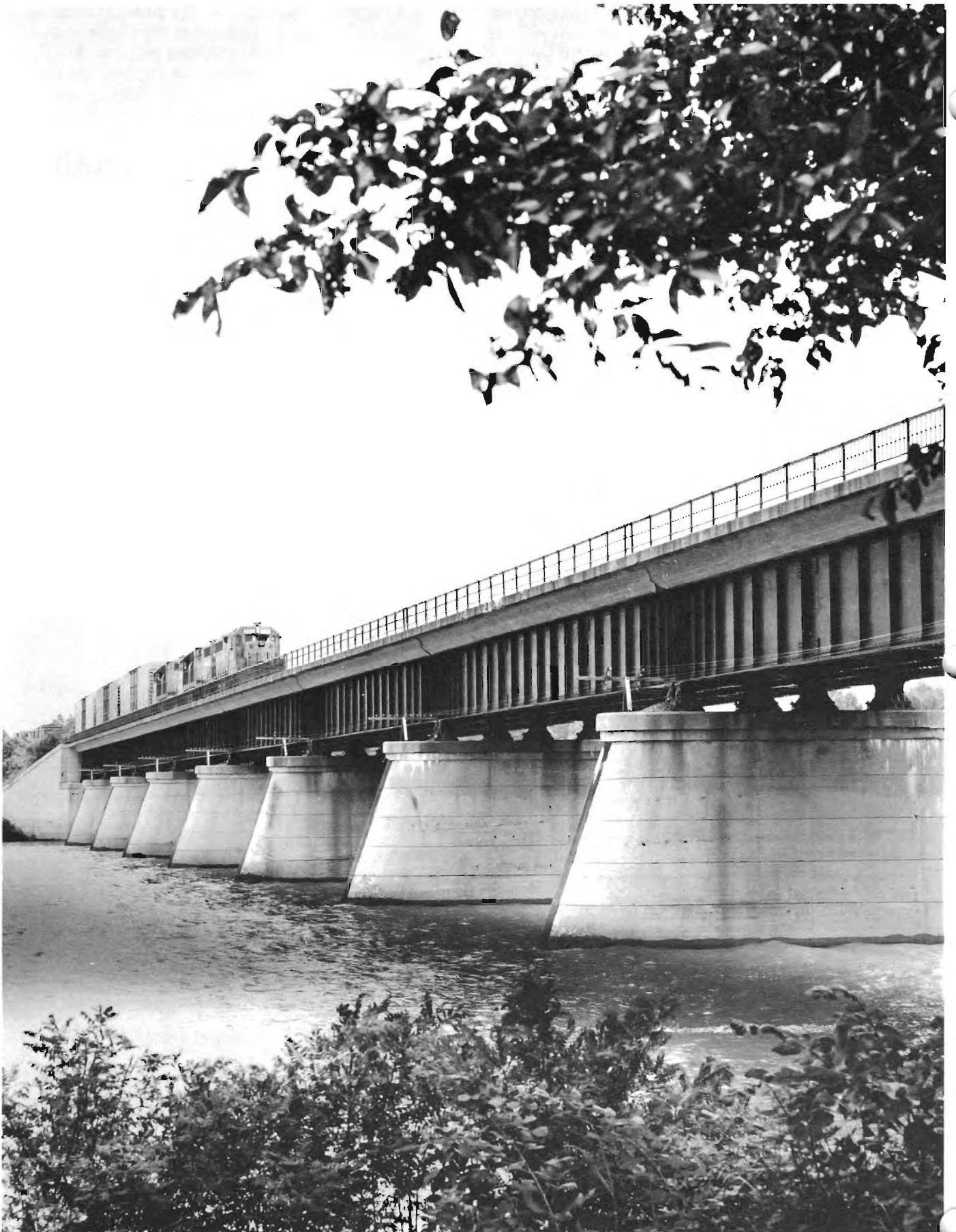
DC-9 bound for Cincinnati and lead by GP-38 205 and two other units crosses the double track bridge over the Maumee River near Napoleon, Ohio on 7/1/79.
